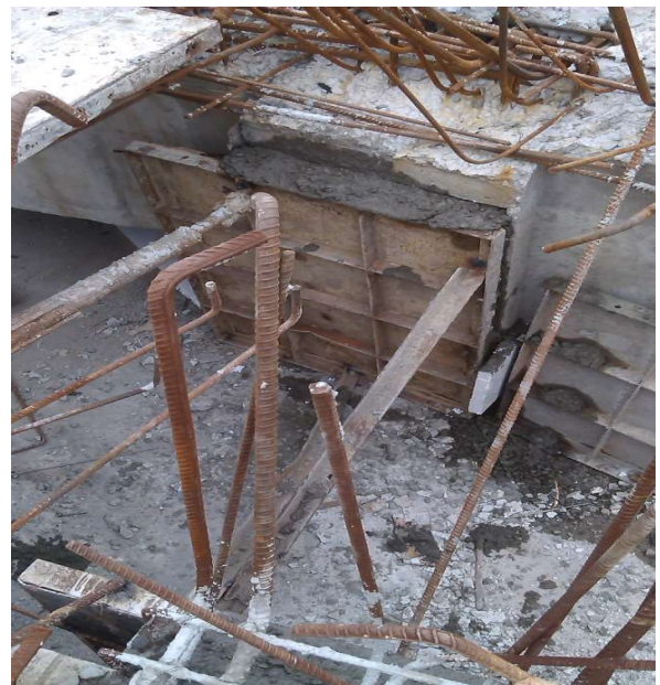
Figure 8 Closing section after prestressing of the beam.
