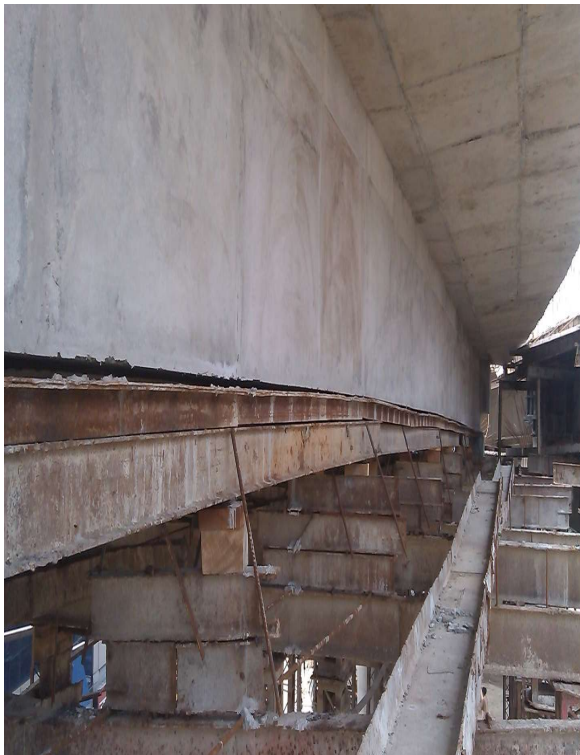
Figure 5 Setup for the prestressing of the beam.
