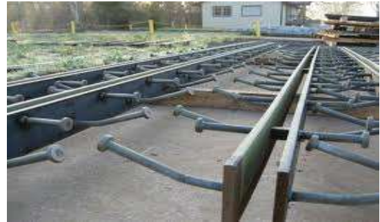
Figure 10 Expansion joint setup
