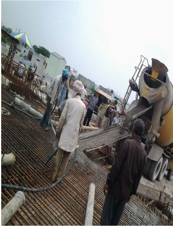
Figure 9 casting of the deck slab of the bridge.
