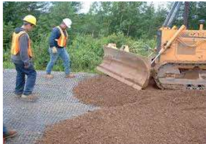
Figure 12 Base course material
