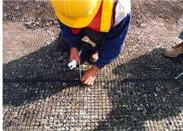
Figure 11 Tie-up of the geogrids.
