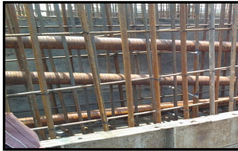
Figure 3 Prestressing cable layouts
