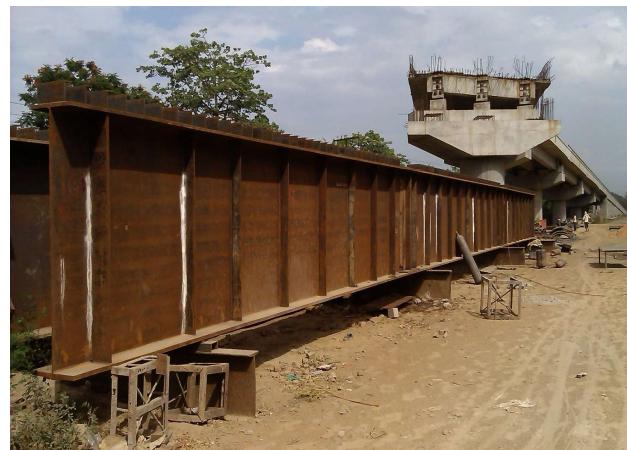
Figure 2 Girder for the railway overhead beam.
