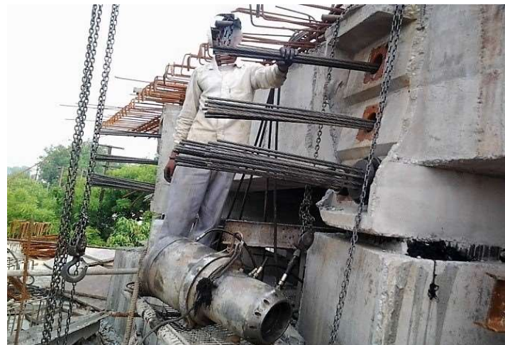
Figure 4 before the prestressing of cable.
